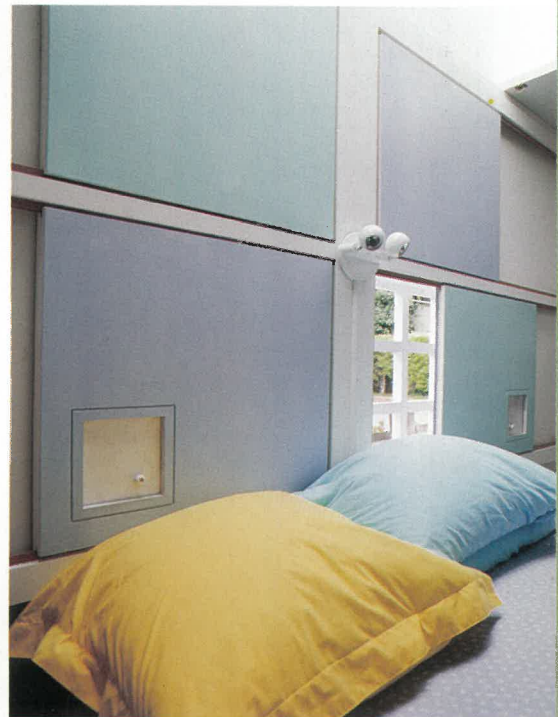
Fresh air. Sliding shutters over the master-bedroom headboard can be opened to take advantage of the breezes on balmy nights. The 2x2 grilles on the outside are security screens. Note the little doors on the lower shutters. They can be opened individually to let in just a little ventilation in cold weather.
