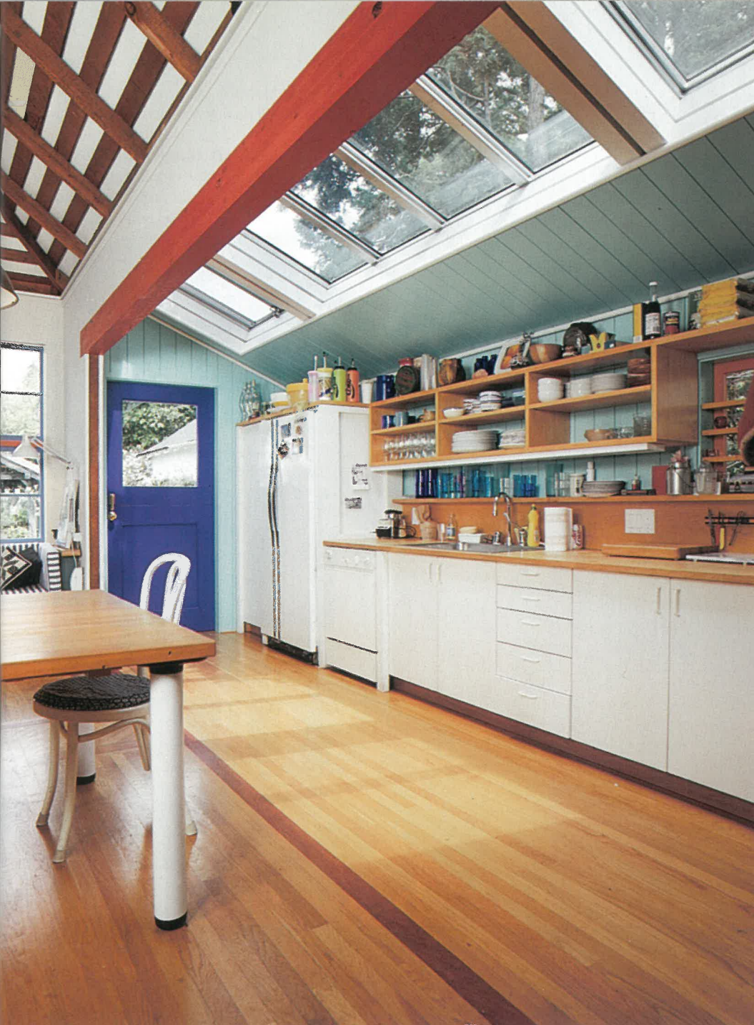
Under skylights. The new kitchen is laid out along a single wall for ease of access. A row of skylights stretches the kitchen's entire length, helping to illuminate the vibrant color scheme. Where old walls have been partially removed, their patches have become inlays in the new oak floor plan. For example, the mahogany strip that recedes toward the door from the bottom of the photo marks the line of the east wall of the original kitchen. In the upper left corner, the original skip sheathing is revealed as the new ceiling finish.
