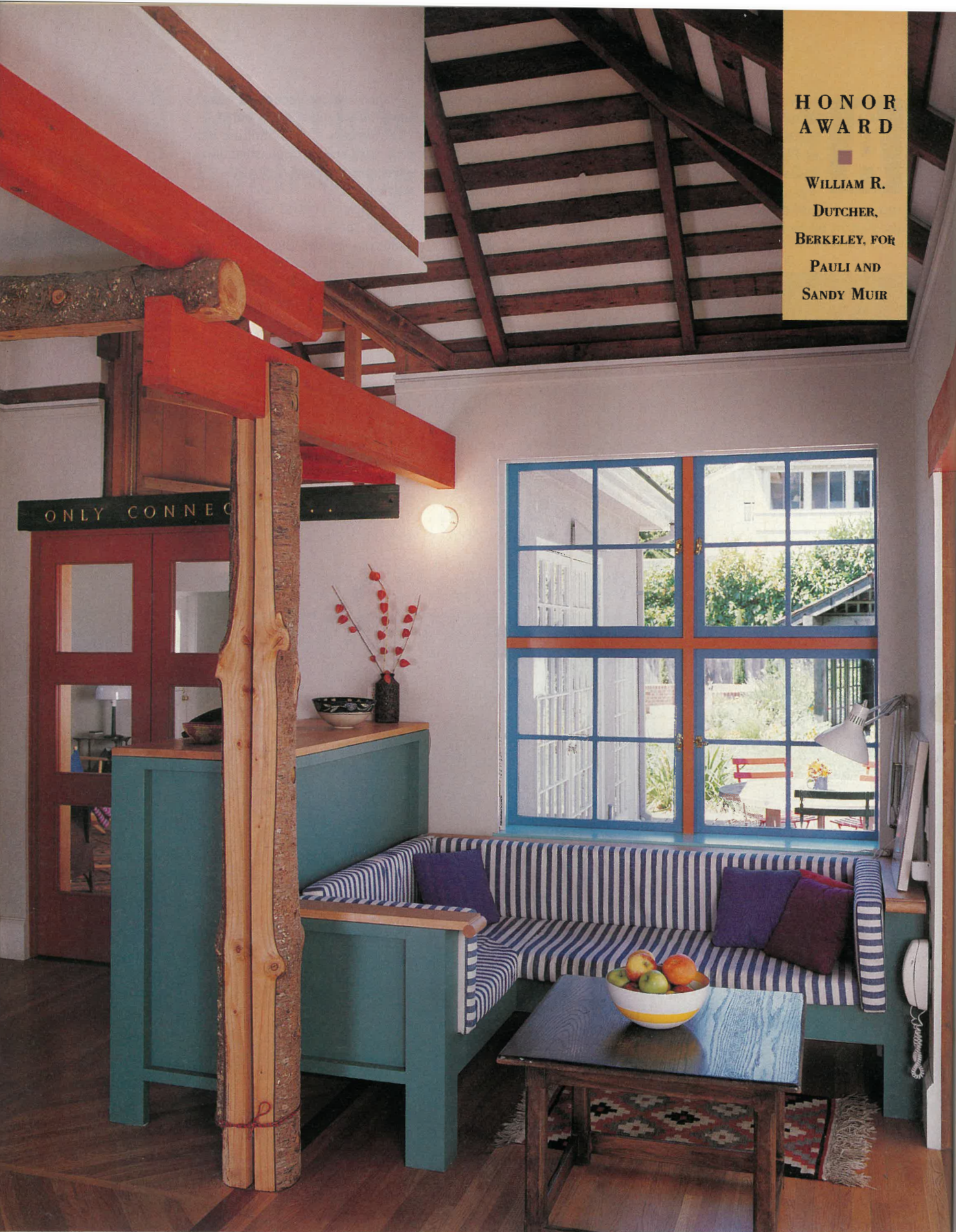
ORANGE-STAINED BEAMS and unpeeled logs sawed flat on two sides replaced load-bearing walls in kitchen area, layering support within open volume.
