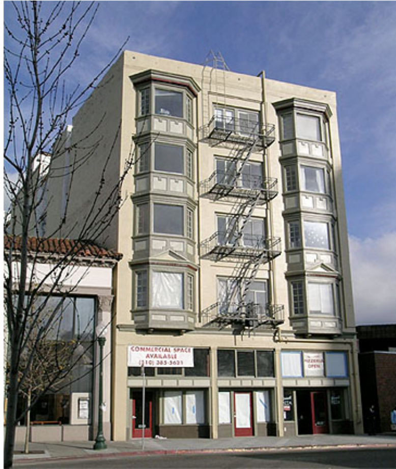
F.D. Chase Building, 2107 Shattuck Avenue (photo: Daniella Thompson, 2004)
