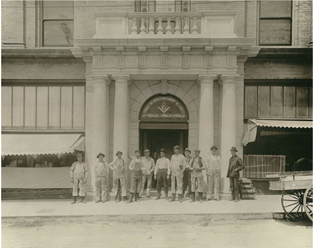
Wharff (4th from r) and the real masons who built the Masonic Temple, 1906. Note the granite pillars, later removed. (BAHA archives)
